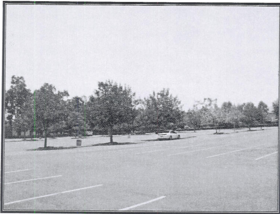
Common Area Parking Lot
