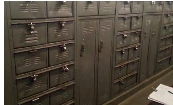
Locker rooms are in need of reconfiguration and additional P.E. lockers.
