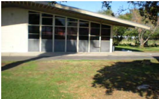
Landscape and irrigation in need of renovation.
