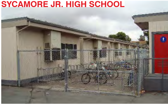
26 portable classroom units to be converted to permanent classrooms.
