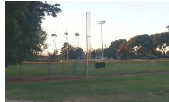
Need to install tall security fencing.
