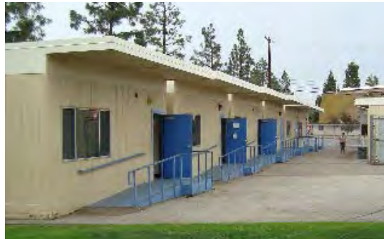
9 QEIA portables will be removed soon. Propose second bus drop off area.
