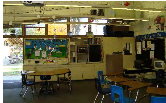
Classrooms require modernization with special needs.
