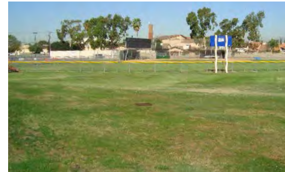
Existing field turf is in poor condition.
