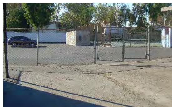
Major improvements are needed in security fencing.
