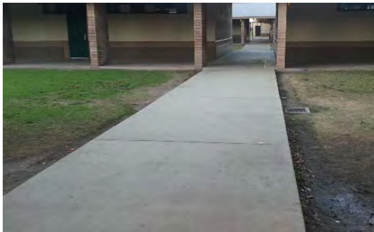
Widen concrete sidewalks.
