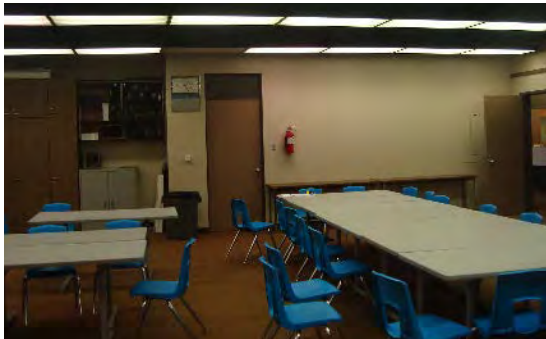
Need to improve lighting.
