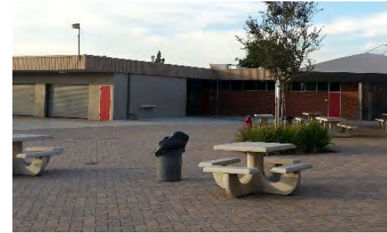
Need new shade structures/lunch shelters.
