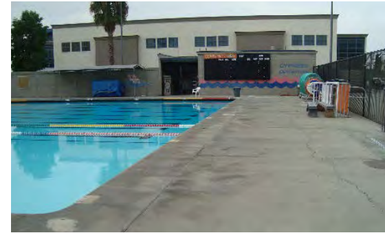
Pool in need of standard modernization.
