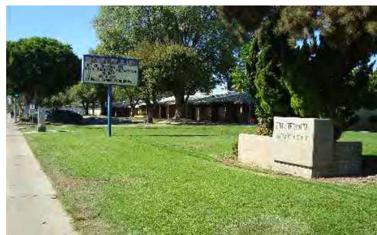
School entrance/site security is in need of redesign.
