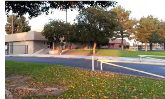
Evaluate the front visitor parking lot.
