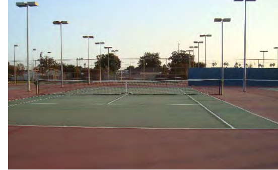
Tennis courts need to be replaced.
