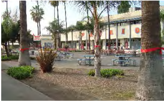
Central quad in poor condition.
