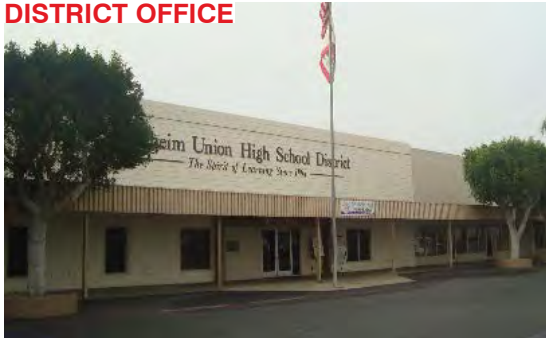
Emphasize main entry to the building.
