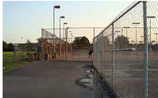
Minor ponding and drainage issues on campus.
