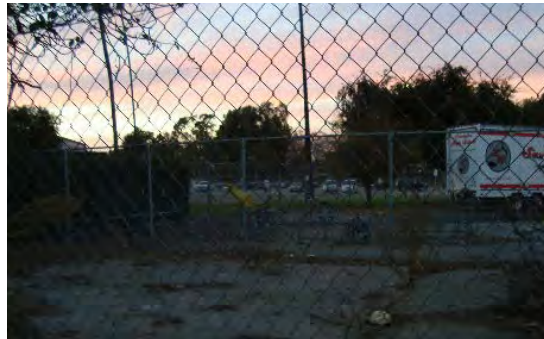
New fencing and security lighting needed throughout campus.
