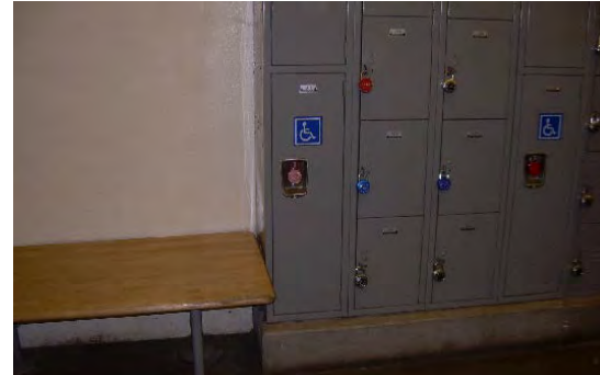
Boys and girls locker rooms need better ventilation.
