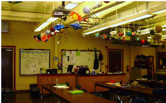
Buildings require major renovation.
