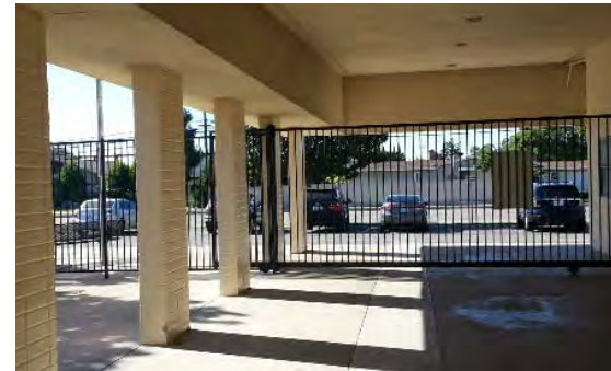
Need to install 8' tall fencing along Ball Road.
