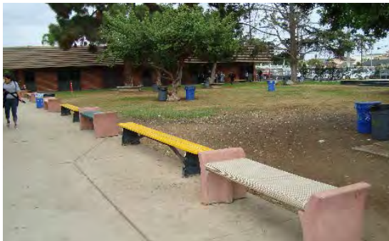
Campus quad in poor condition.
