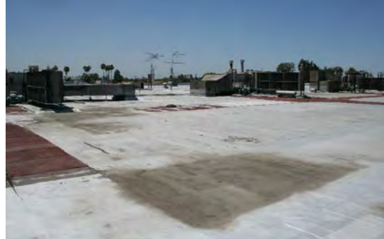
Replace roofing and HVAC units.
